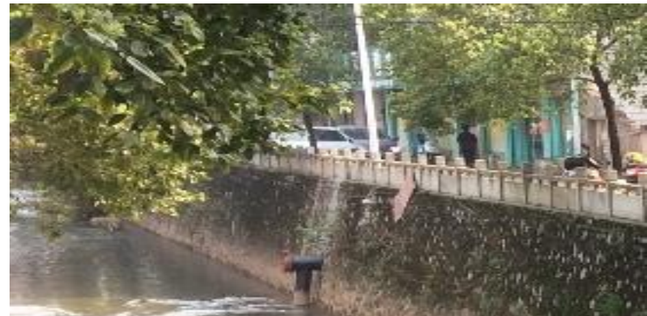
After: all sewage outfall were controlled and reformed
