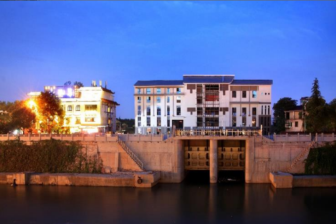
Ehu Pump Station, 60m 3 /s
