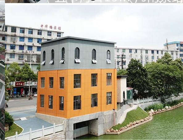
Flood Diversion Sluice
