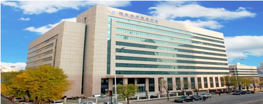
New look after energy-saving reconstruction in September 2016
